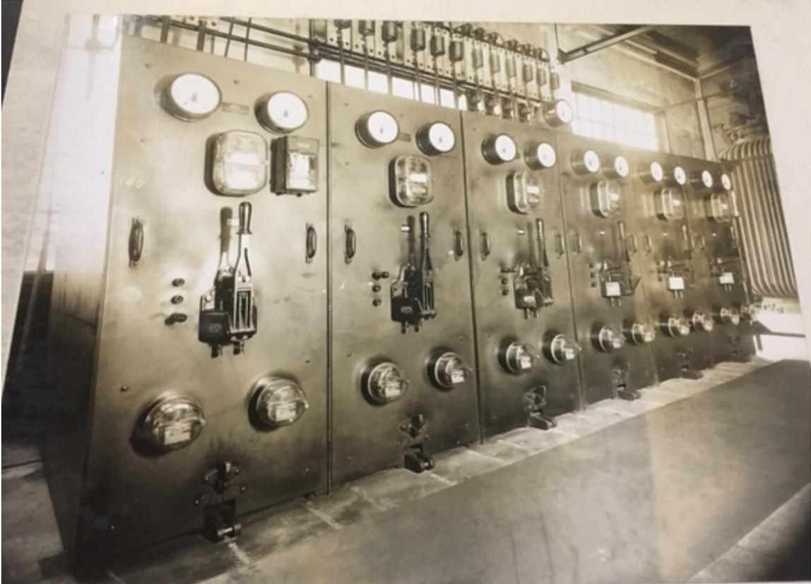
Figure 4 View of the 2.3 kV circuit breakers on the East wall at #10 Substation<sup>9</sup>
