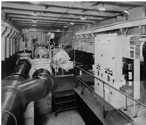
Figure 25: 4 ½ Level Underground pump room at Hazleton Shaft showing twin 10,000 GPM centrifugal pumps
